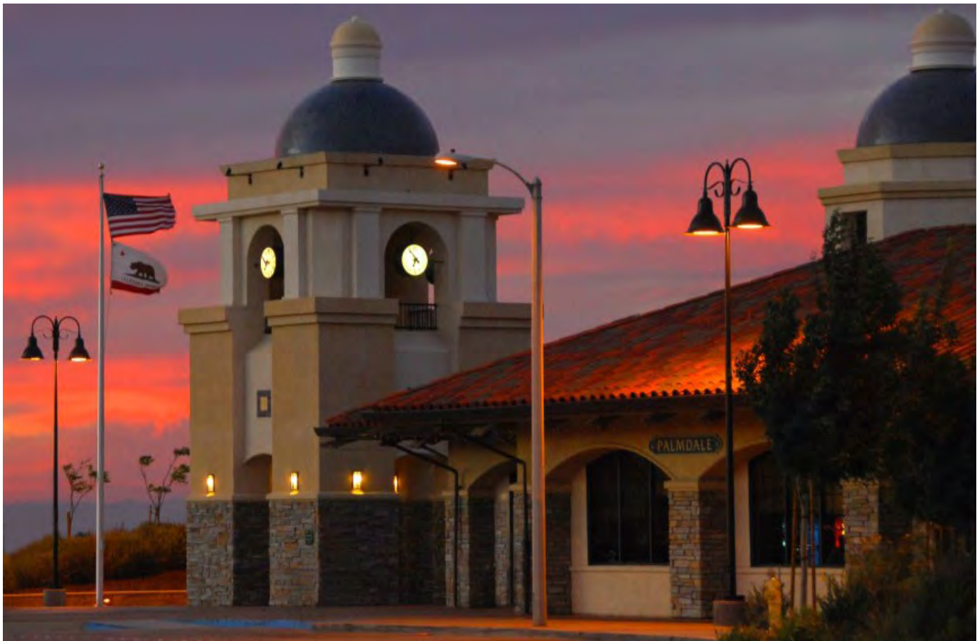
[Contributed image of the Palmdale Transportation Center.]
